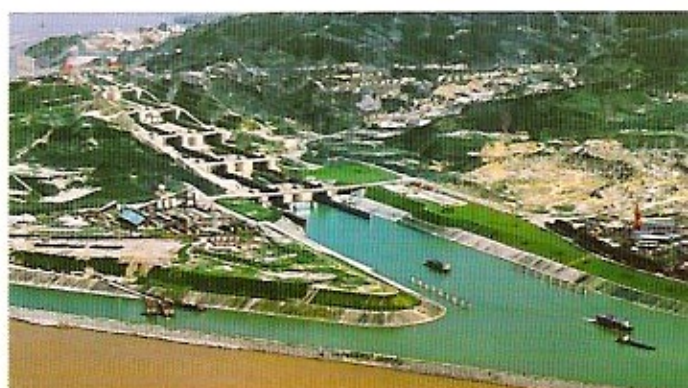
Permanent five-stage ship lock of the Three Gorges Project
